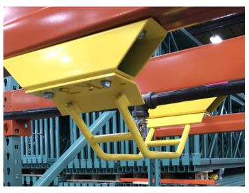
K3 In-Rack Sprinkler Guards are made for ultimate protection. Other sprinkler guards that attach directly to some component of your sprinkler system (pipes, fittings, or sprinkler head) can be easily broken and dislodged by heavy machinery, causing severe damage to your sprinkler system. K3 Sprinkler Guards attach to the beams, resulting in safer protection for your sprinklers and your entire system.
